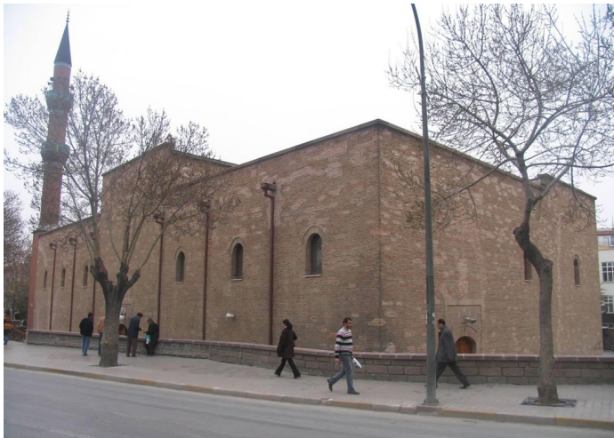
Figure 3. Today's photo of the building.
