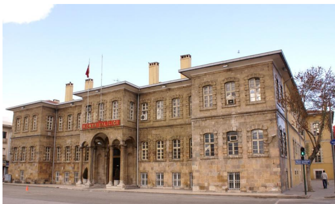
Figure 5. Today's photo of the building.
