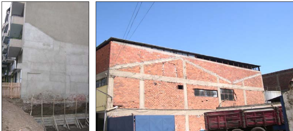
Figure 3. A 5-storey building without a foundation in Şemikler, İzmir (left), an illegal apartment built with the removal of the roof in Çınarlı (right) (Photos; Anonymous, 2009)
