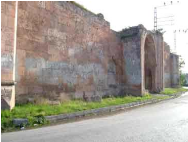
Picture-2; Tokat - Pazar Mahperi Hatun Caravanserai Main Entrance Facade (Foundations General Directorate-Tokat District Directorate)
