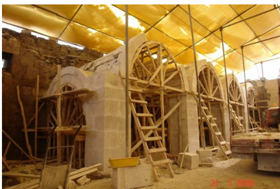
Picture- 8; Tokat - Pazar Mahperi Hatun Caravanserai Closed Court Pendentive Manufacture
