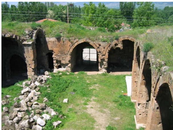
Picture-4; Tokat - Pazar Mahperi Hatun Caravanserai Open Inner Court (Foundations General Directorate-Tokat District Directorate)
