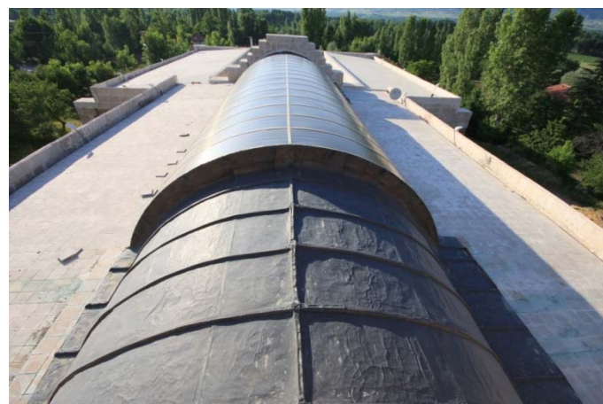
Picture-15; Tokat - General View of the Pazar Mahperi Hatun Caravanserai Roof
