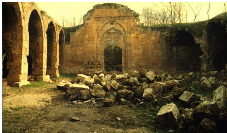
Picture-6; Tokat - Pazar Mahperi Hatun Caravanserai Open Inner Court (Foundations General Directorate-Tokat District Directorate)
