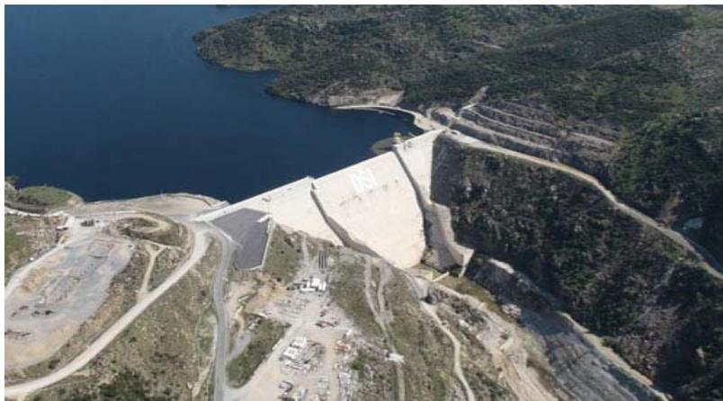
Fig. 1. Cine Roller Compacted Concrete Dam
