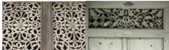
Fig. 7. Tebuk tembus to facilitate ventilation.
