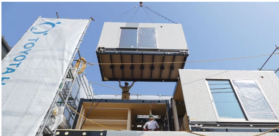
Figure 3. Module fabrication at Toyota
